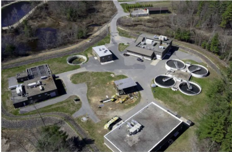
A wastewater treatment plant in Maine. PFAS chemicals have been linked to cancer. Cj Gunther/EPA, via Shutterstock
